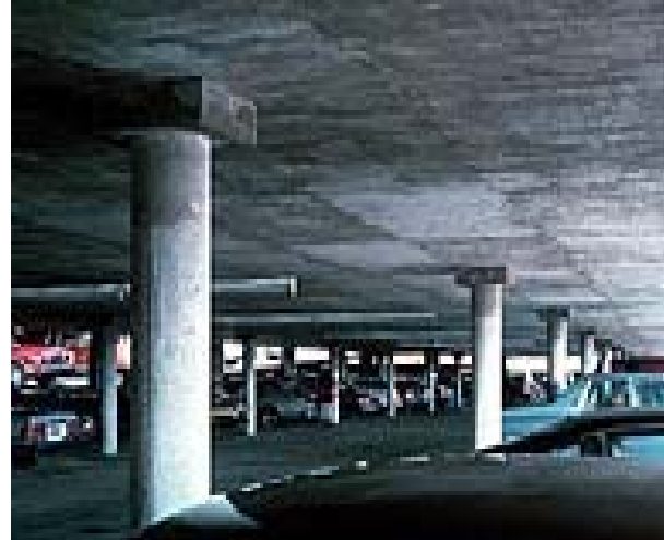
Figure 4: Flat Plate W/ Drop Panels
